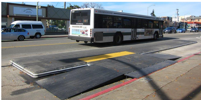
Figure 1: Example Temporary Bus stop Infrastructure
